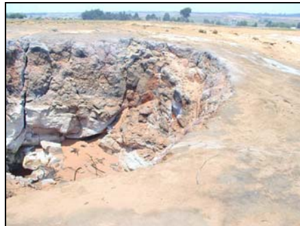
Figure 2. Surface collapse due to abandoned burning workings at T&DB.
